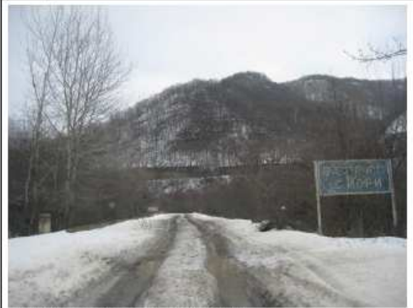
Iori River crossing at km 3.3
