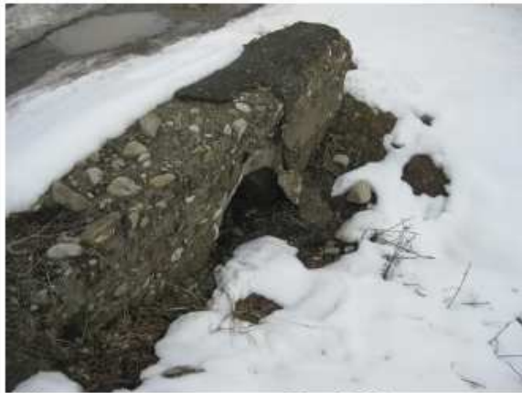
Culvert under access road, km 0.95
