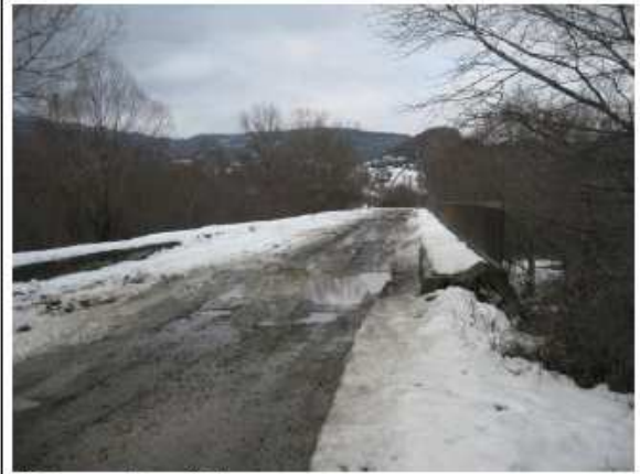
Bridge at km 2.1
