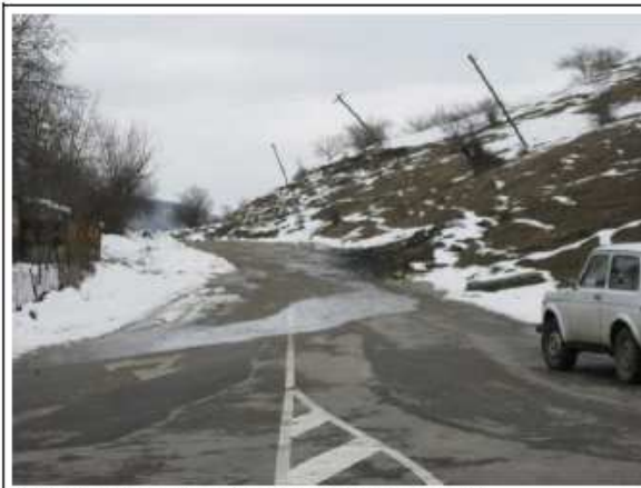
Beginning of the Project Road, km 0
