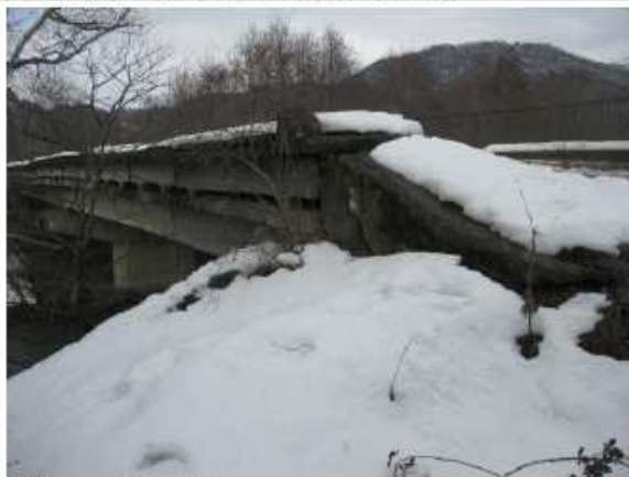
Bridge at km 2.1
