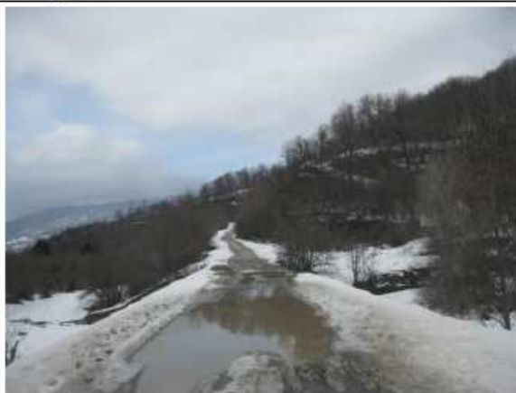
Road at km 3.9
