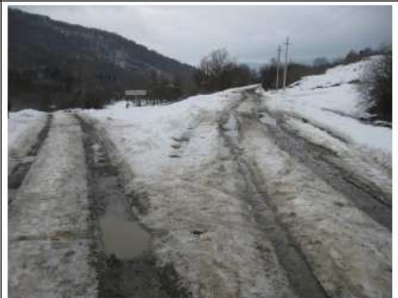
End of the Project Road, Junction
