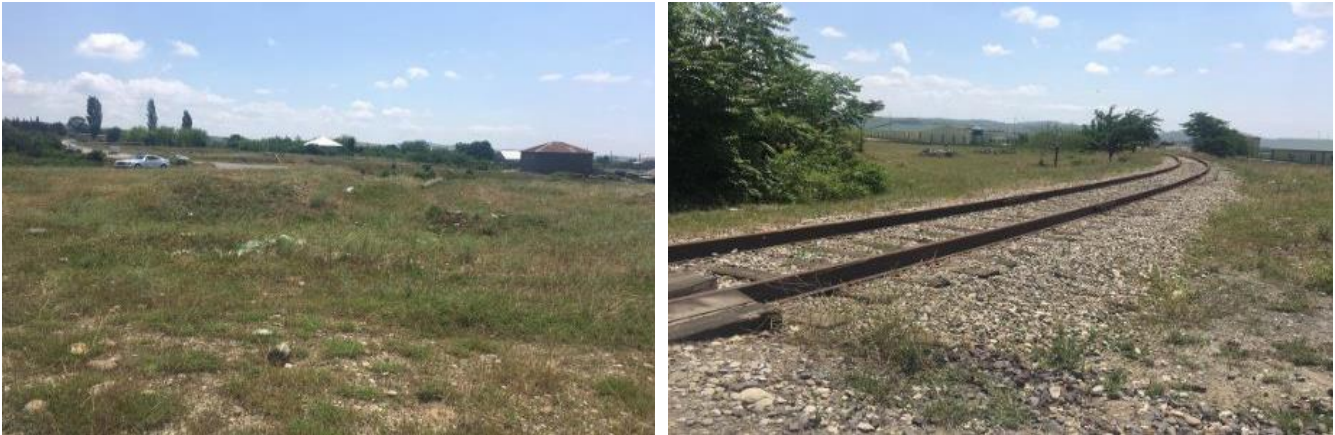
Photo 6.2.4 General views of the corridor near village Kachreti
