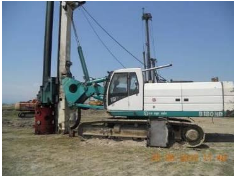
Picture 2.1 Drilling Equipment Widely Used for Pile Arrangement in Georgia
