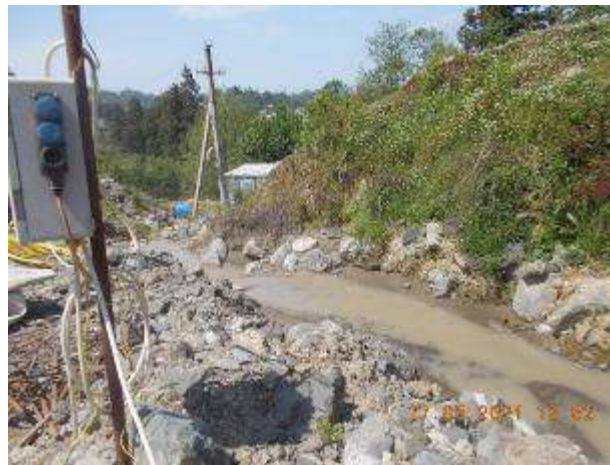
Photo 54 T3 sedimentation trap
