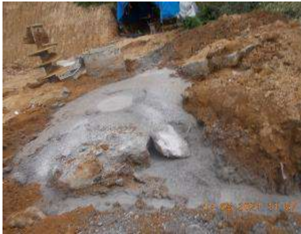
Photo 41 T2 Leaked concrete
