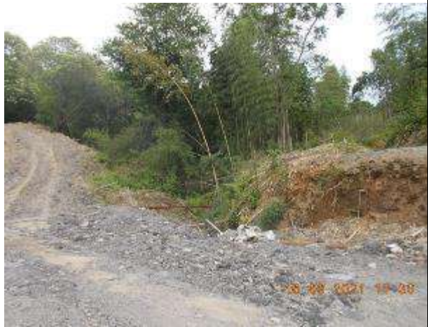
Photo 62 T1 Cut Bamboo waste
