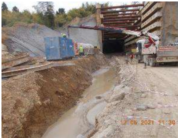
Photo 53 T2 sedimentation trap
