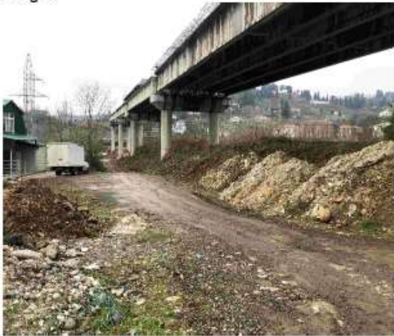
Photo No. 7- Excavated soil and rock material placed under bridges
