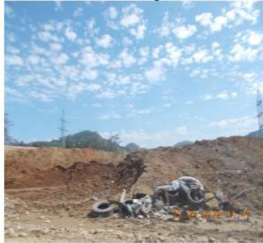
Photo No. 8- Near the Interchange No. 4.
