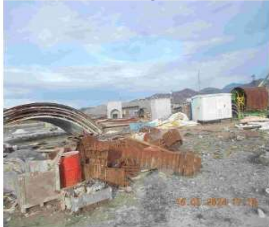
Photo No. 2- Construction camp site
