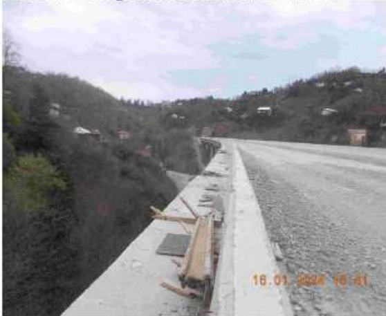
Photo No. 5- Bridge No. 10 shoulder and sidewalk
