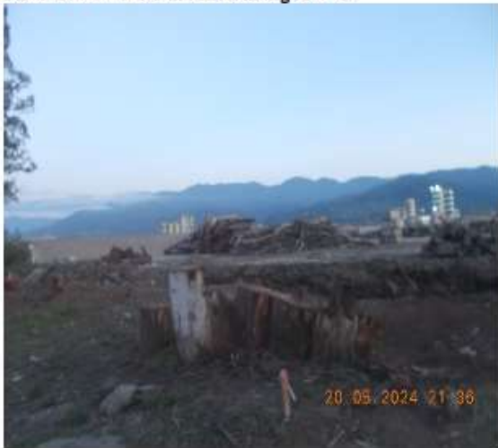
Photo No. 9- Near the Interchange No. 4.
