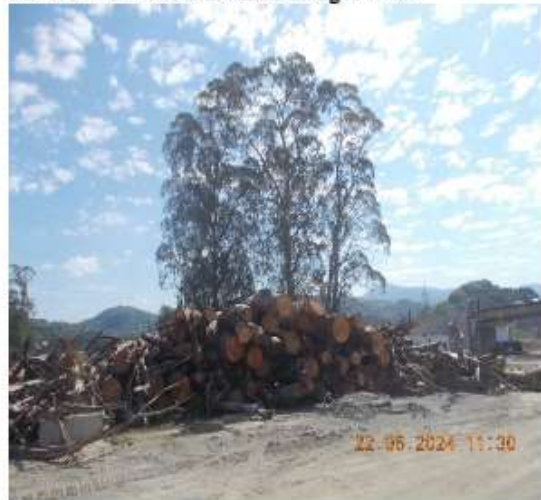
Photo No. 10- Near the Interchange No. 4.
