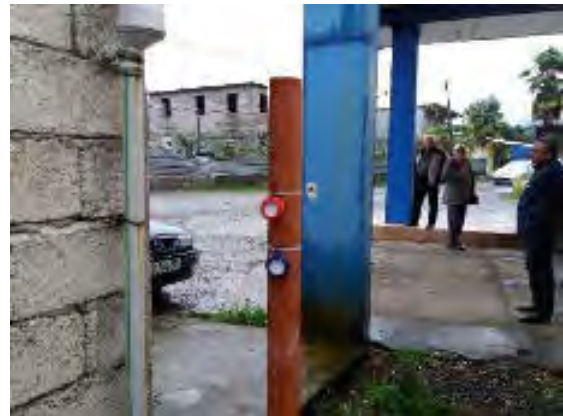
Rapid Air Monitors at A3
