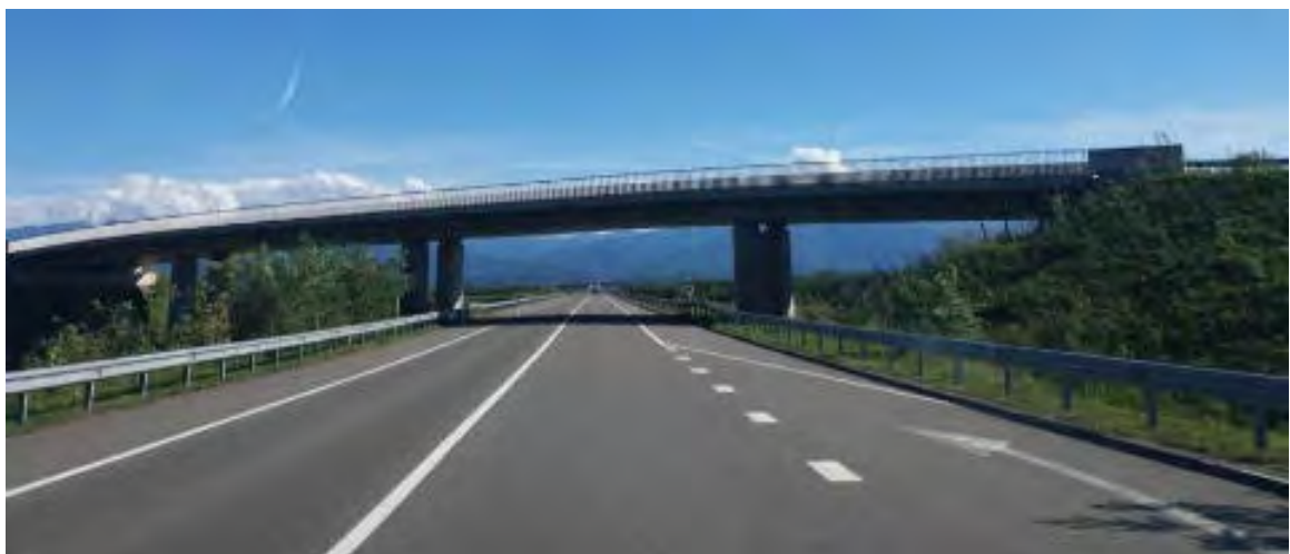
Figure 1-4: A Bridge over Kobuleti Road with Similar Design
