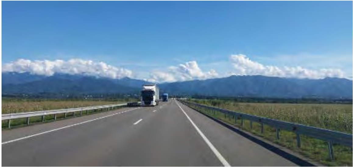
Figure 1-2: Kobuleti Bypass Road
