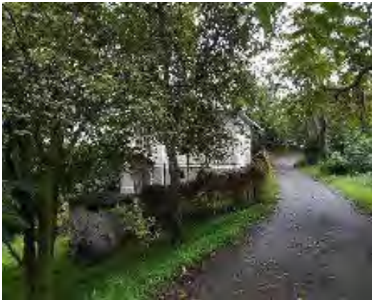
Freshly asphalted road.
