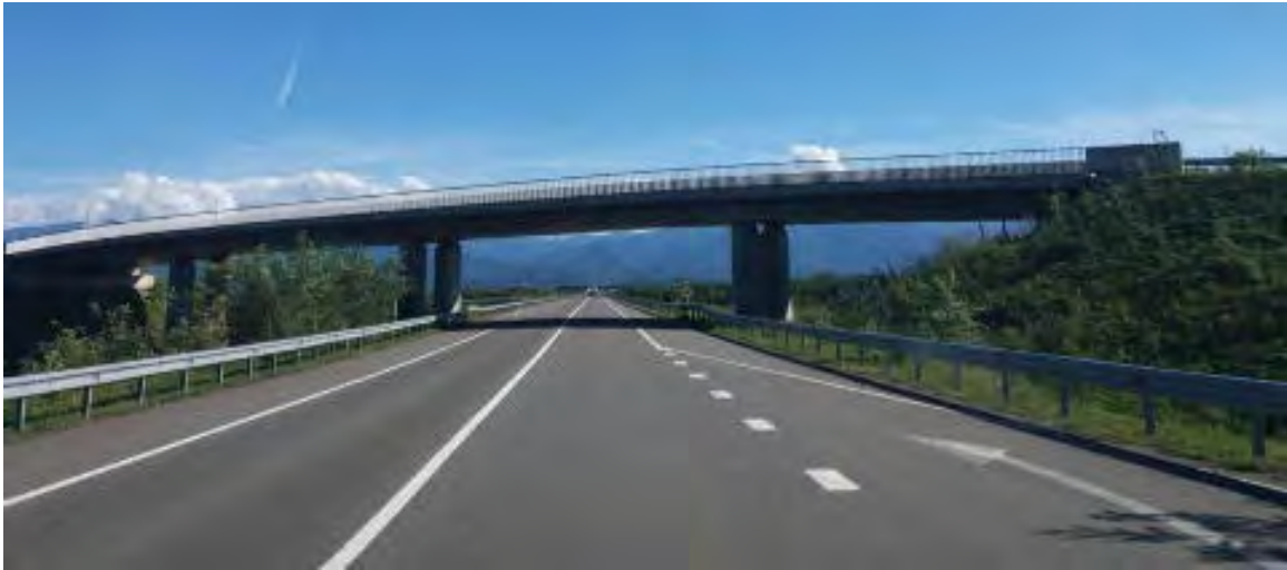
Figure 4-14: A Bridge over Kobuleti Road with Similar Design
