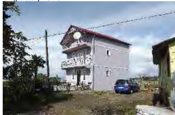
New doubly story structure
