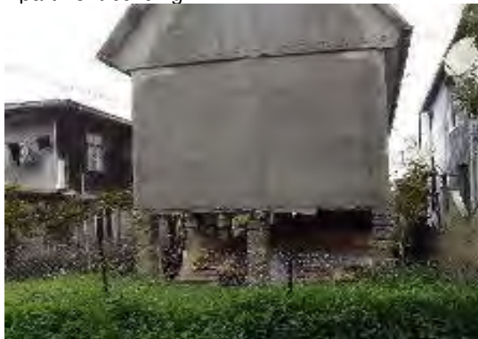
House constructed with blocks as foundation
