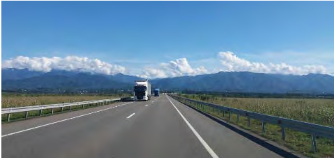
Figure 4-4: Kobuleti Bypass Road
