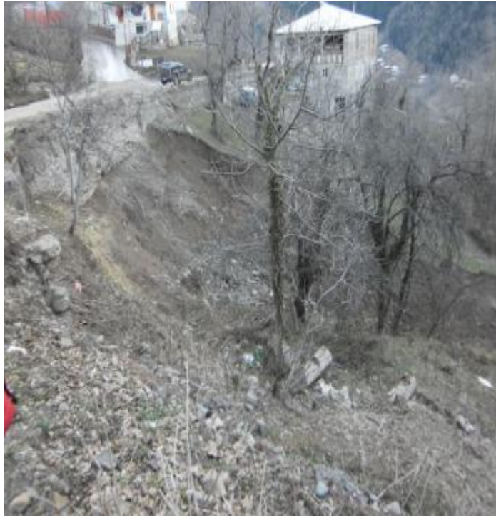
Pic 4.5 Current Situation on Landslide District (km 0+400)
