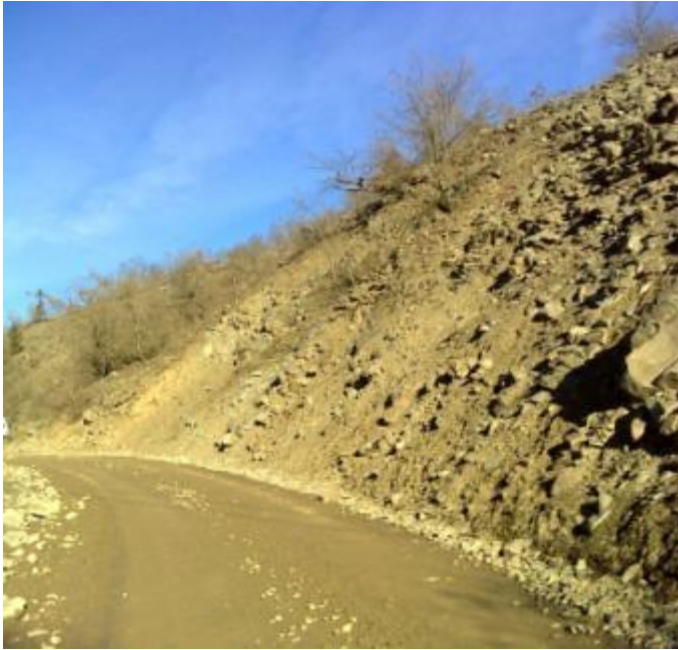
Pic. 4.7 Steep Slope Ripped Off Stones and Rocks
