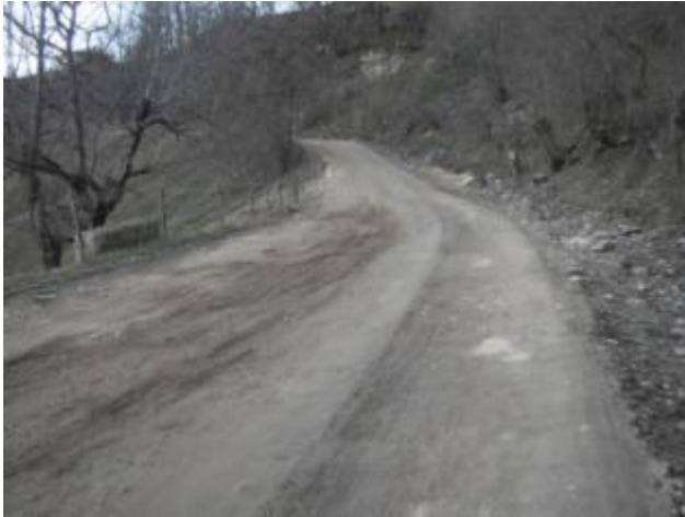
Pic. 4.6 Damaged and Repaired Districts of the Road
