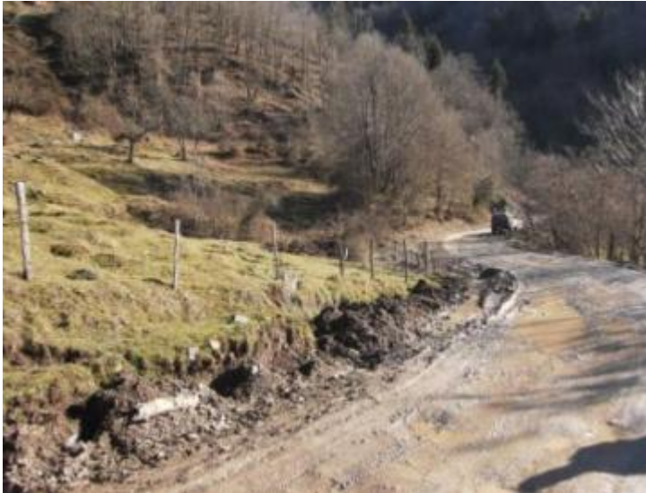
Pic. 4.8 Landslide N2 (km from 5+560 to km 5+620)
