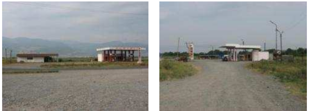
Figure 6.1 Non-residential buildings along the Ruisi - Agara road section
