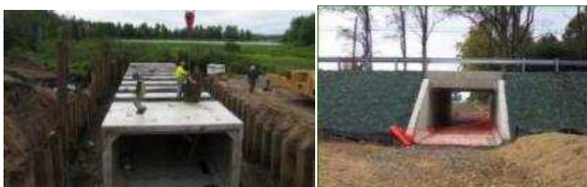
Figure 4.7 Construction of the crossing as a, simple box culvert underpass
