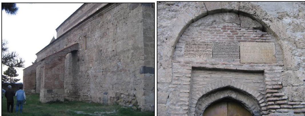
Pic. 6.5: Sioni Church of Urbnisi
