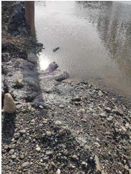
Cement Residues in the River on the Peninsula
