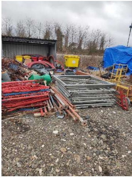
Hazardous waste storage area
