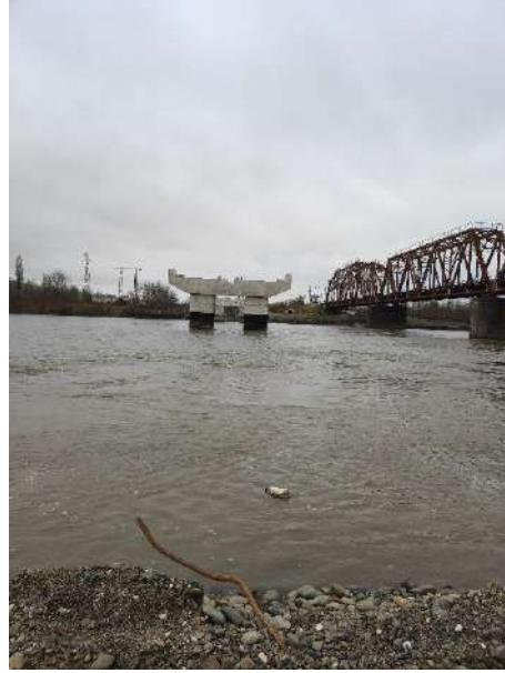
Panoramic view of the bridge pier location near the Rioni river
