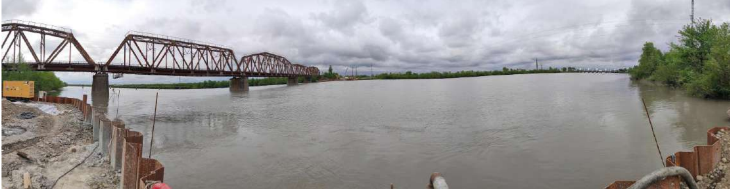
Panoramic view of the bridge pier location near the Rioni river
