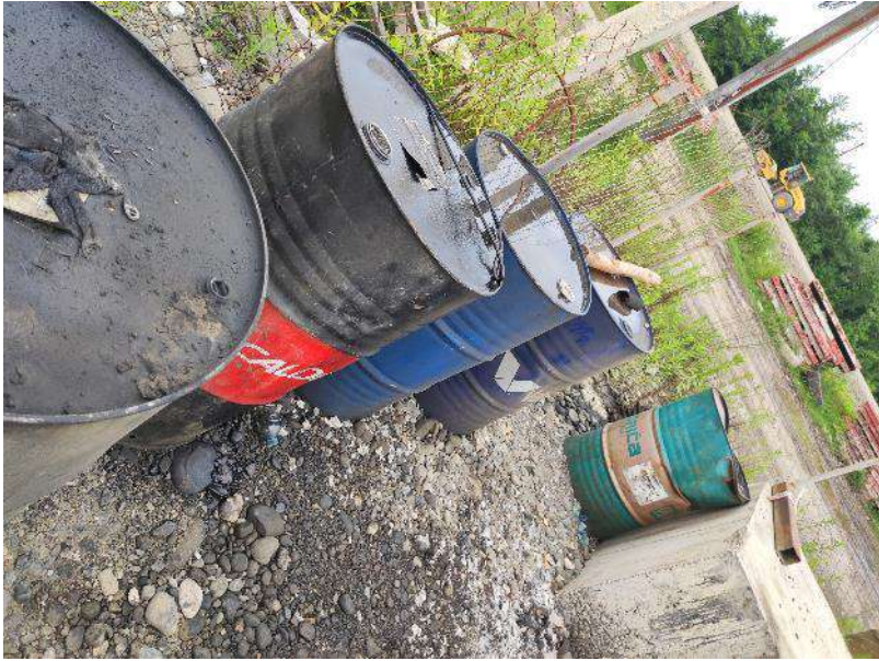
Improperly stored hazardous waste
