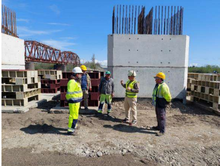
Some Photos from H&S and Environmental Trainings
