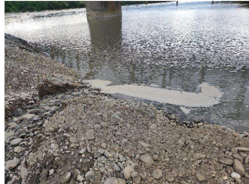
Wastewater Spill into the River from the Peninsula
