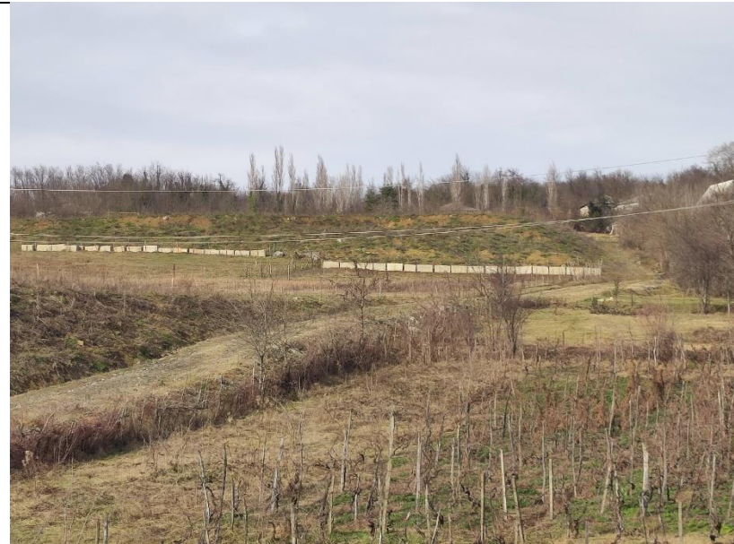
Temp Spoil Disposal 1
