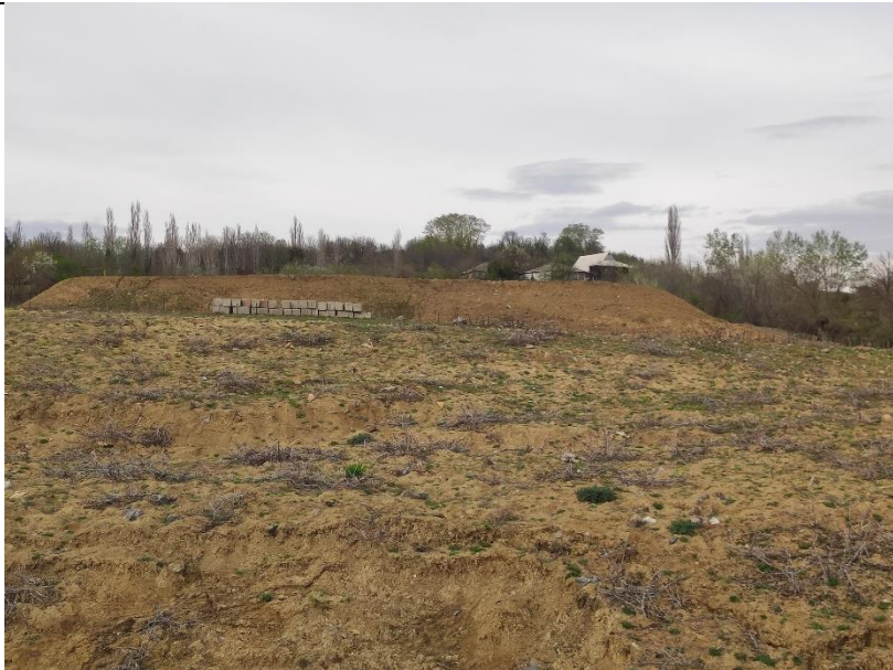
Temp Spoil Disposal 1
