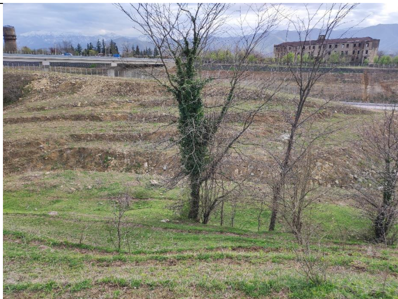
Drainage Channel Structure for Spoil Disposal Site 3
