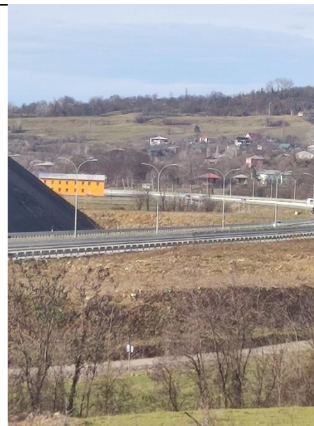
Temp Spoil Disposal 2/1 – 2/2
