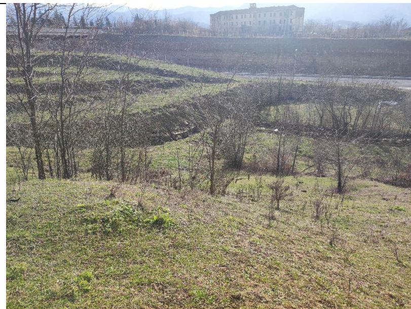
Drainage Channel Structure for Spoil Disposal Site 3
