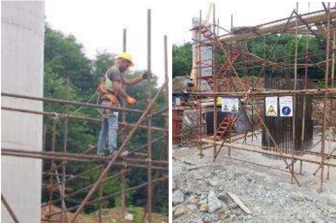
Picture 21: Non-compliance (Work at height-possible fall) (Bridge #5) - Workers have been caught in unsafe position during working at height. They were equipped with personal body harness, but weren't connected to the pipe supports. Actually, they should fix themselves to the scaffolding pipe, to avoid possible falls, but they did not do it. Work activity was suspended for a few minutes. The Engineer asked workers to use body harness properly and fix themselves to the structure and avoid possibility of falling and only after that continue perform the job. After discussion finish, helpers wear the body harnesses on, fixed it to the scaffolding pipe and only after that continue performing the task. Later on, special warning signs, informing workers about the procedure on how to use the scaffold structure, have been fixed on. Issue closed.
