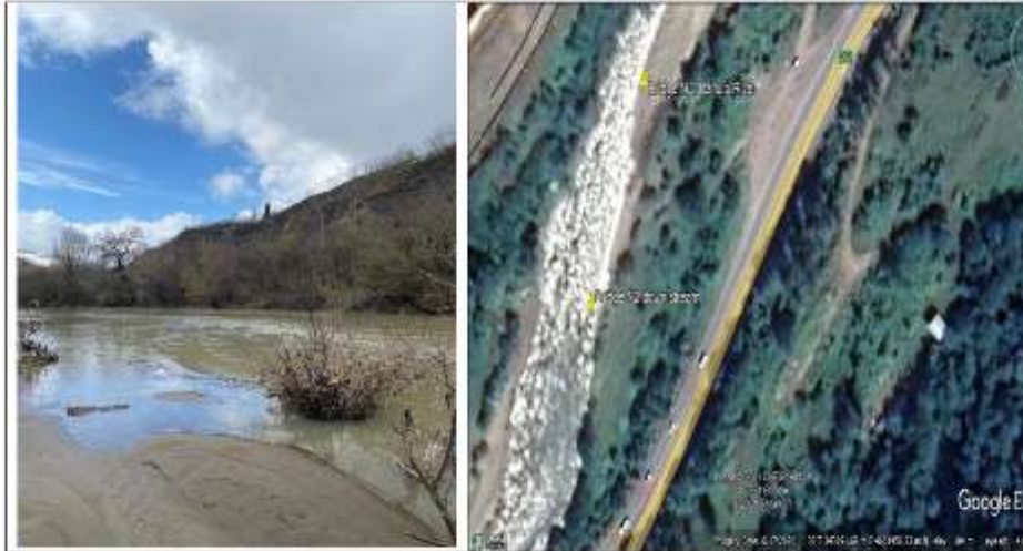
Figure 5-6 Bridge N2 downstream (Dzirula River)
