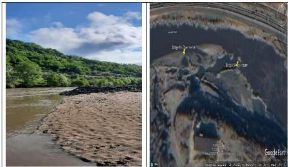
Figure 5-1 Bridge N4 up stream (Kviria River)
