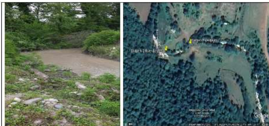
Figure S-3 Bridge N3 upstream (Dorimelo River)
