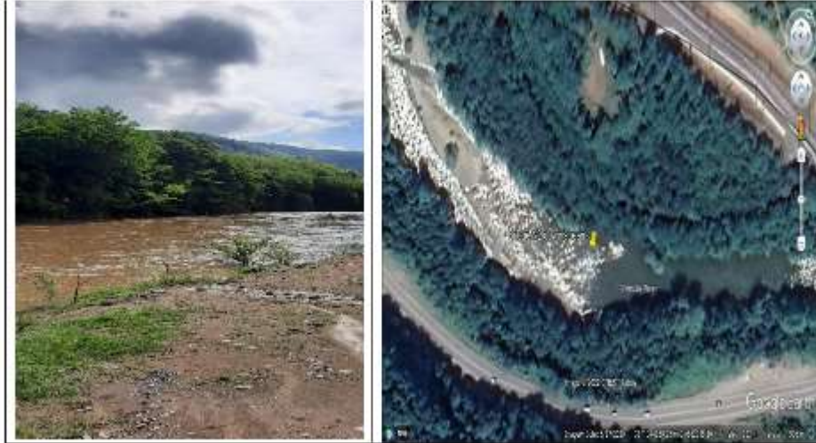
Figure 5-2 Bridge N1 downstream (Zinula River)
