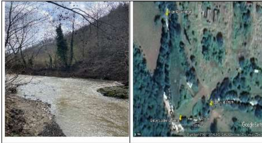
Figure 2-4 Bridge N1 downstream (Kinnemla River)
