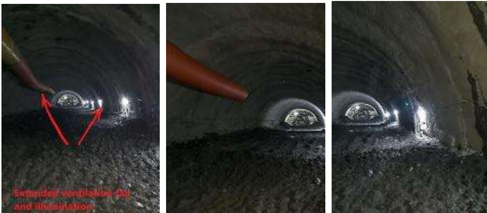
Picture 7: Non-compliance (Poor ventilation and lighting) (Tunnel N3) –During visiting the tunnel a few days ago, it was observed that the ventilation fan wasn't extended to sufficient length and lighting bulbs were missing too. Contractor's site responsible persons were informed by the Engineer. The Engineer asked to pay additional attention on such issues to avoid possible incidents at workplaces. After few days, the ventilation fan was extended and additional illumination bulbs have been installed Issue closed.
