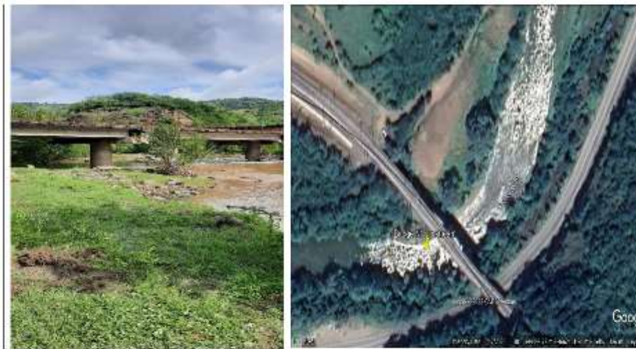
Figure 5-7 Bridge N1 up stream (Dzirula River)
