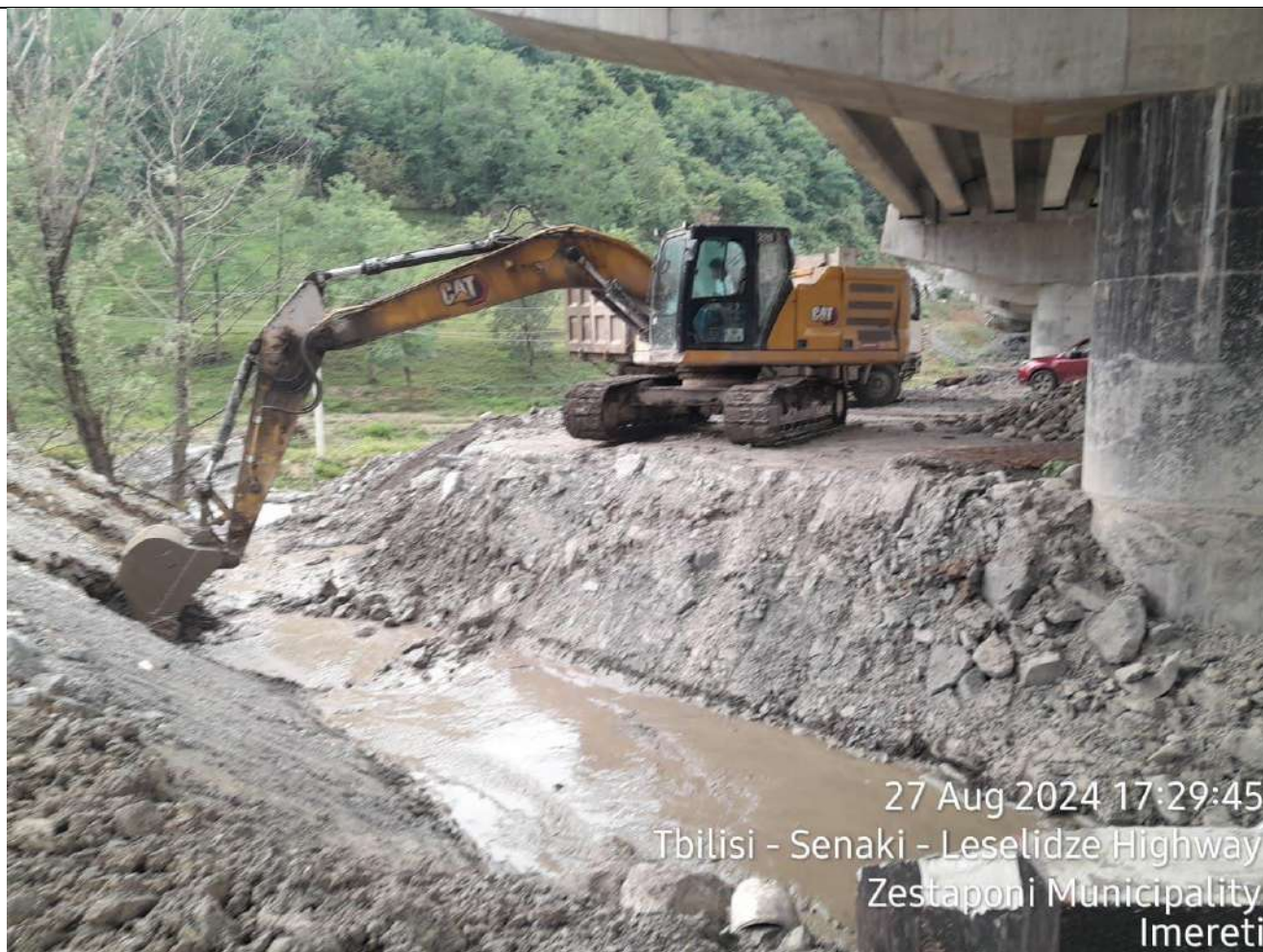
Batching Plant Temporary Sediment Trap Construction (August 2024)
