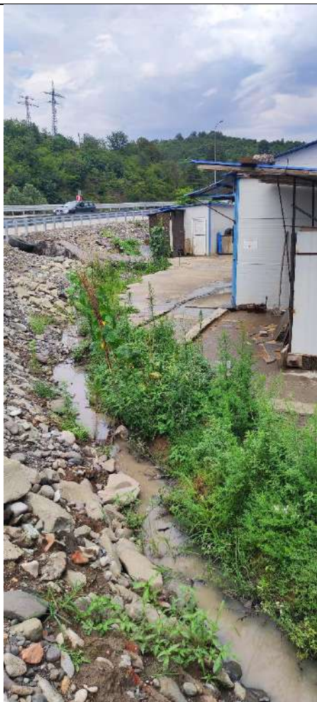
Leaking Sewage Tank (Worker's Camp No 3, July 2024)
