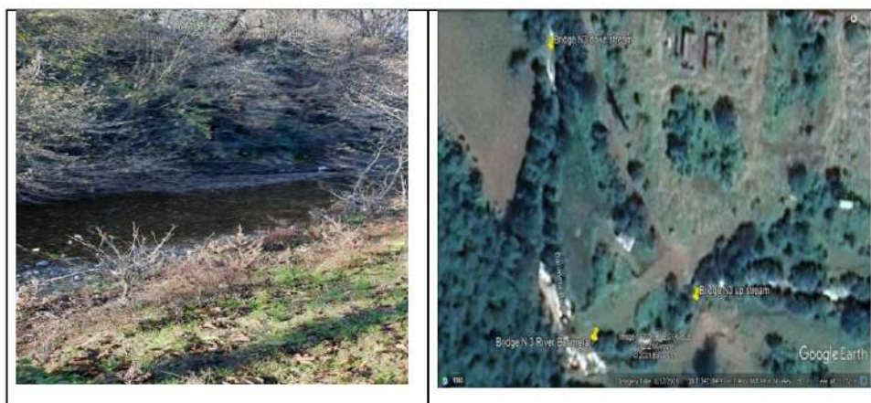
Figure 5-2 Bridge N3 downstream (Borimela River)
