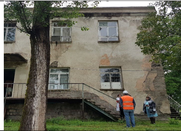
Meeting with population of village Puti living on the top of the Tunnel 3 to inform them about the results of vibration survey conducted by the order of Department under the construction of Shorapani-Argveta section (F4) of E-60 international highway
