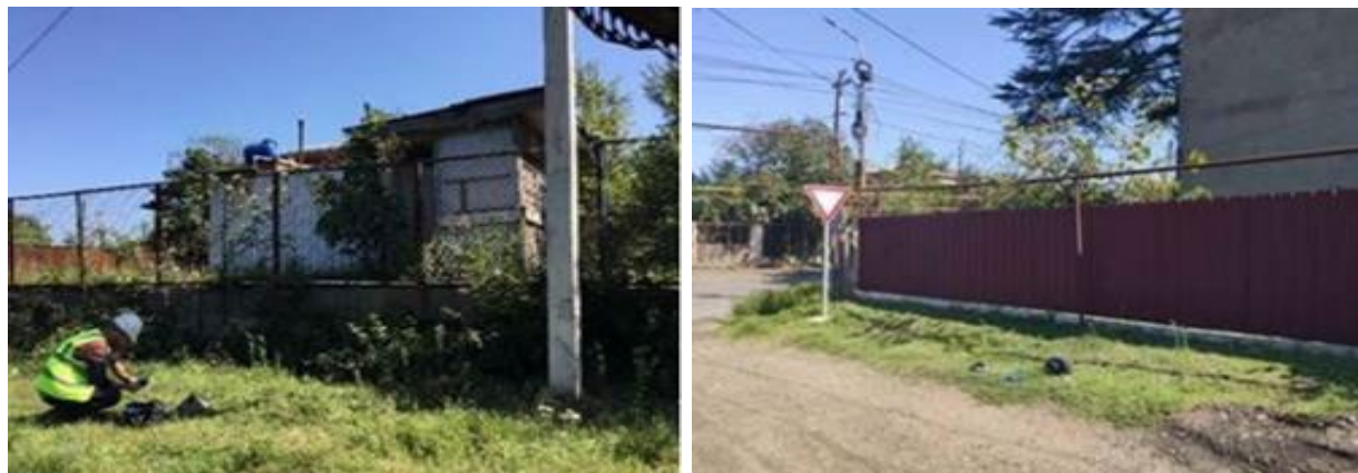
Figure 5: A View of Vibration Monitoring Activities in the Month of September 2021
