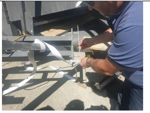
Improper anchors for the dust collectors
