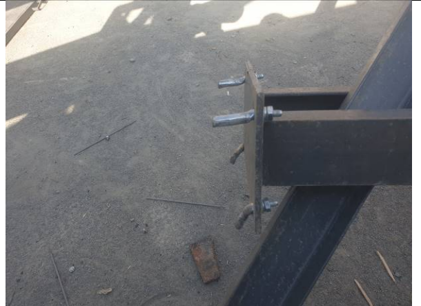
Improper anchors for the dust collectors
