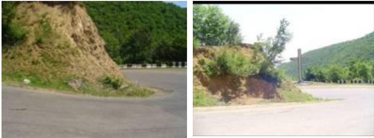
Figure 4-6 Turnings that needs to be improved.
