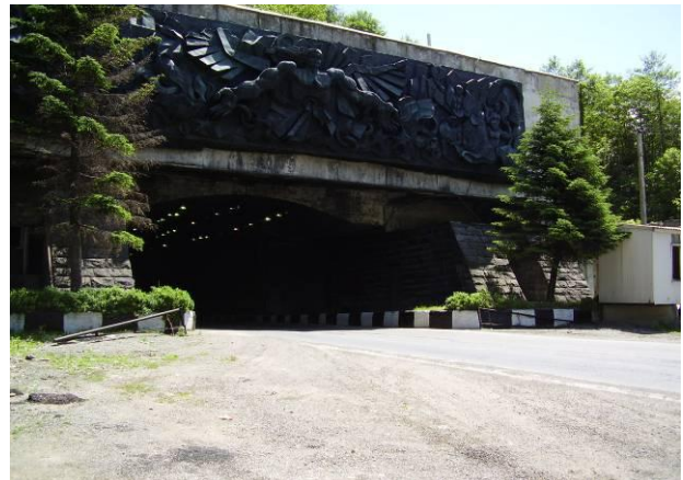
Figure 4-2: Western tunnel face of the Rikoti Tunnel
