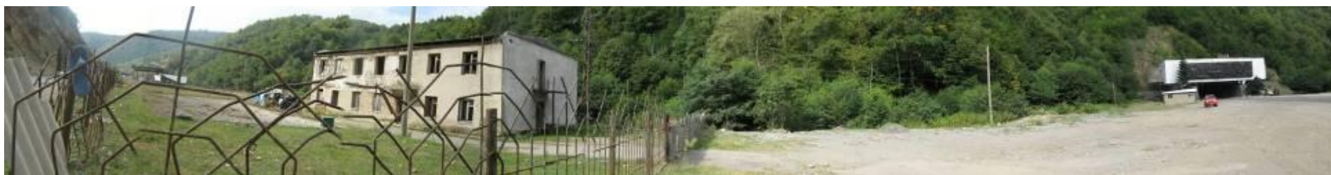
Figure 8-2. Eastern tunnel portal: potential worker's camp and space for concrete batch and/or asphalt mobile plant location.
