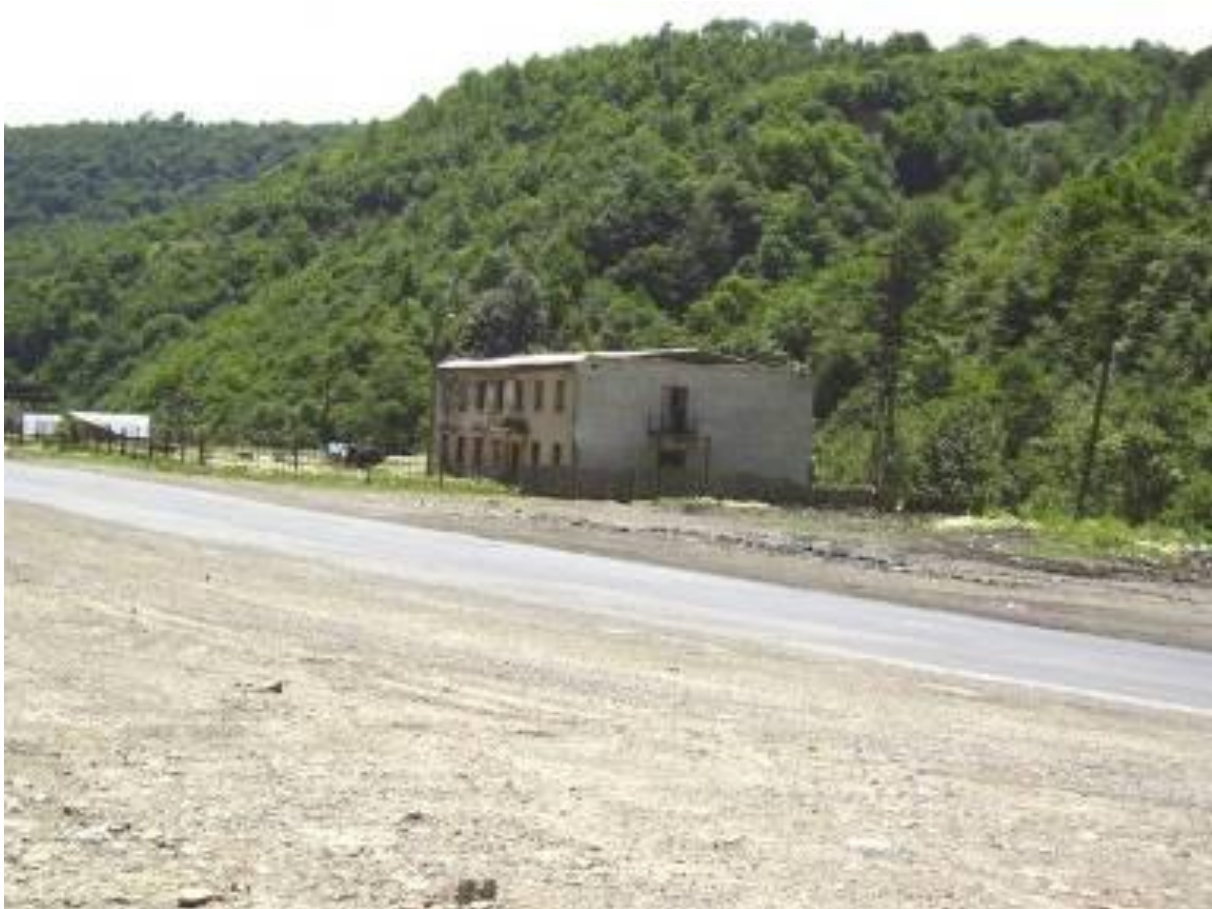
Figure 4-9 The building in the vicinity of the tunnel.
