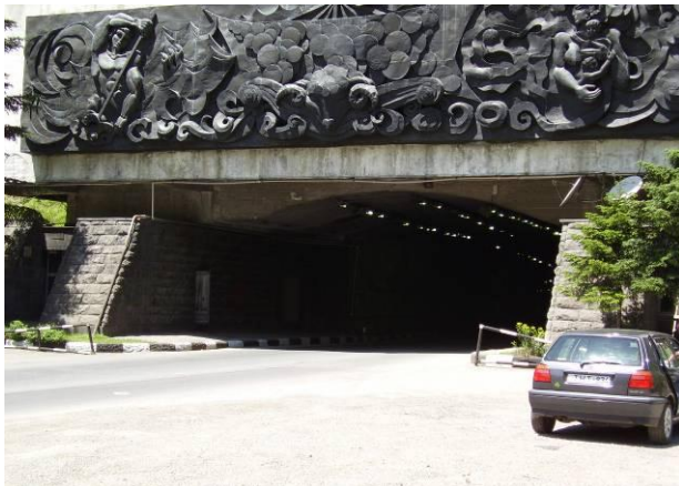
Figure 4-1: Eastern tunnel face of the Rikoti Tunnel.
